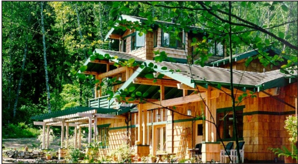
The Shingle Style derived home demonstrates appropriate massing, material palette and detailing.
